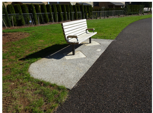
Sample of ADA-compliant bench on accessible route with companion space..
