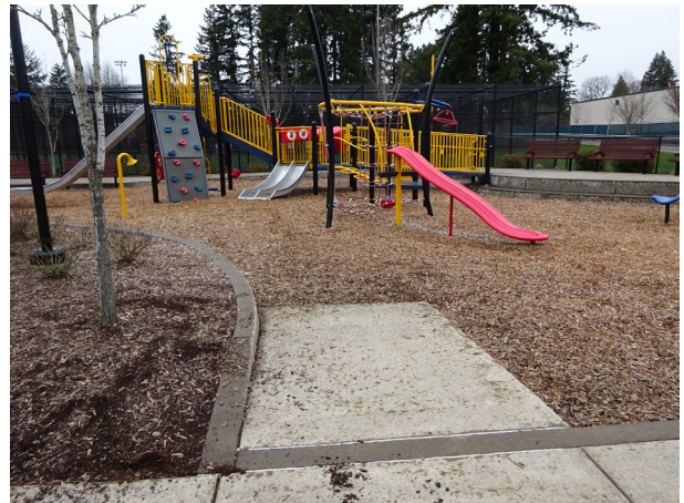
Sample of playground ramp providing access to play safety surface.
