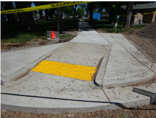
Figure 4. Tactile warning strip
