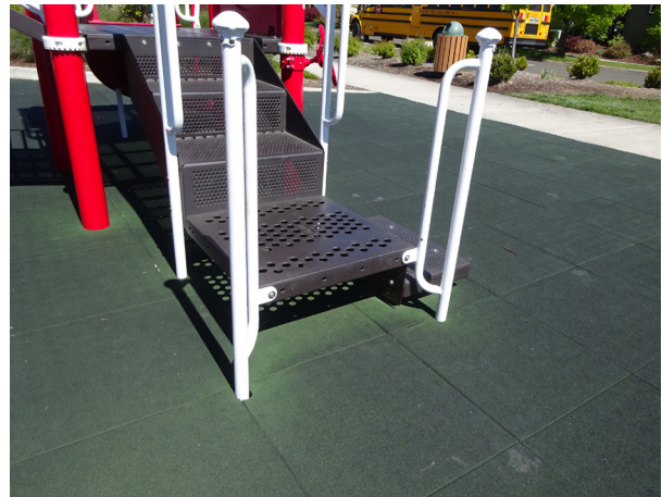
Figure 6. Play equipment transfer platform
