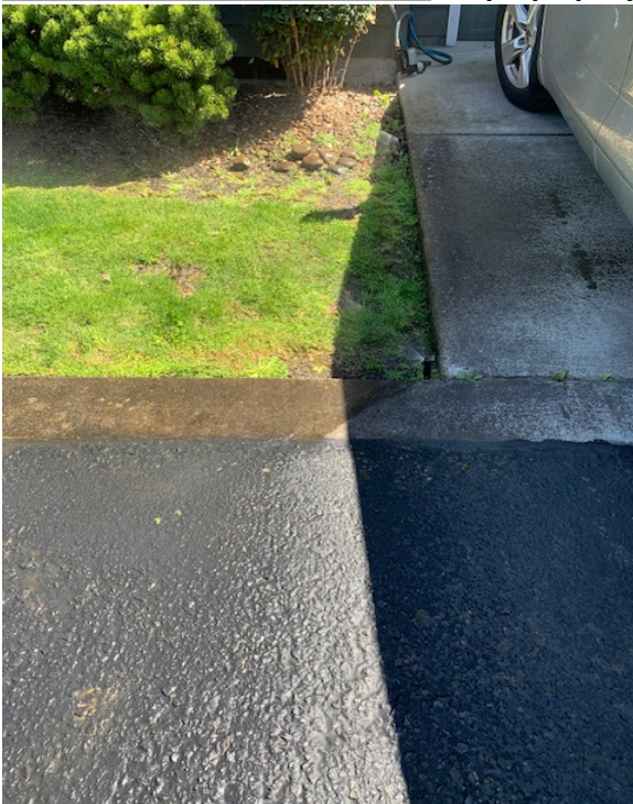
💧 Misaligned Heads watering asphalt. 💧 Broken Emitters
