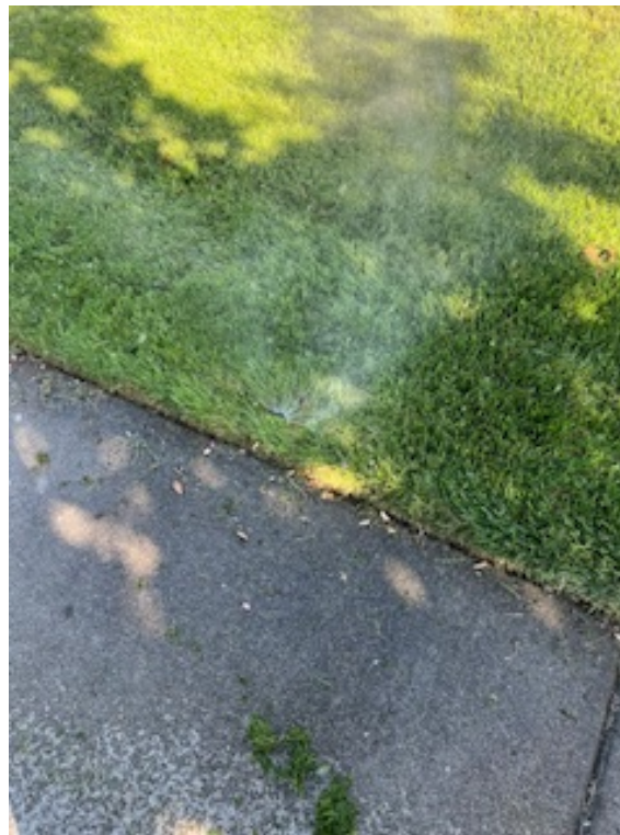
Blocked Sprinkler Head]
