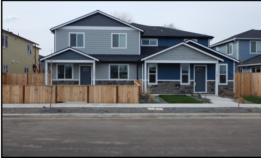
Front view of a finished attached single-family dwelling (two units).
