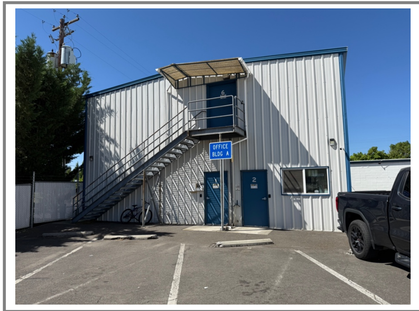
View of rear elevation of office building
