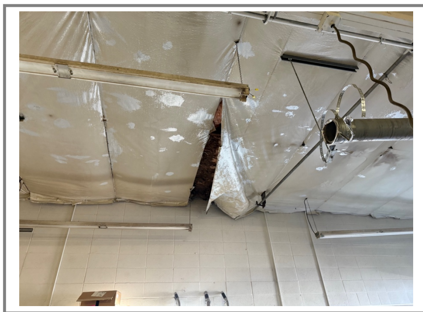
View of ceiling in north side shop building
