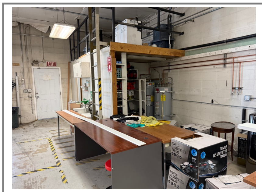
View north side shop mechanical and mezzanine area
