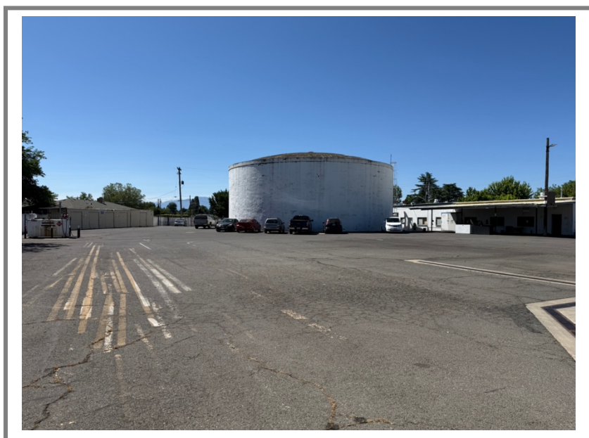
View south across parking lot toward water tower
