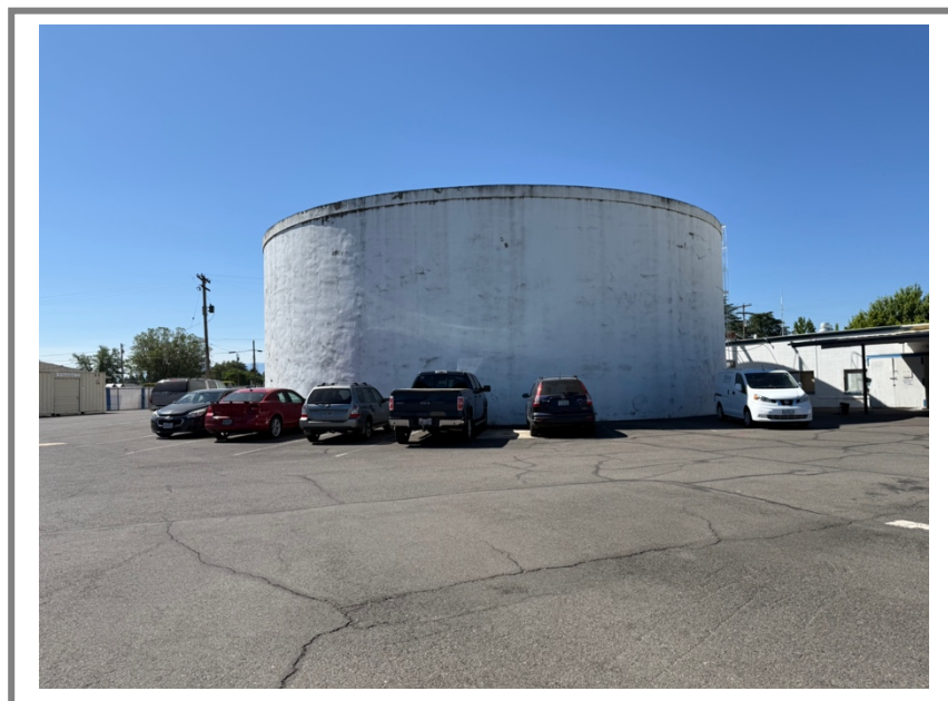
View of parking spaces next to water tower
