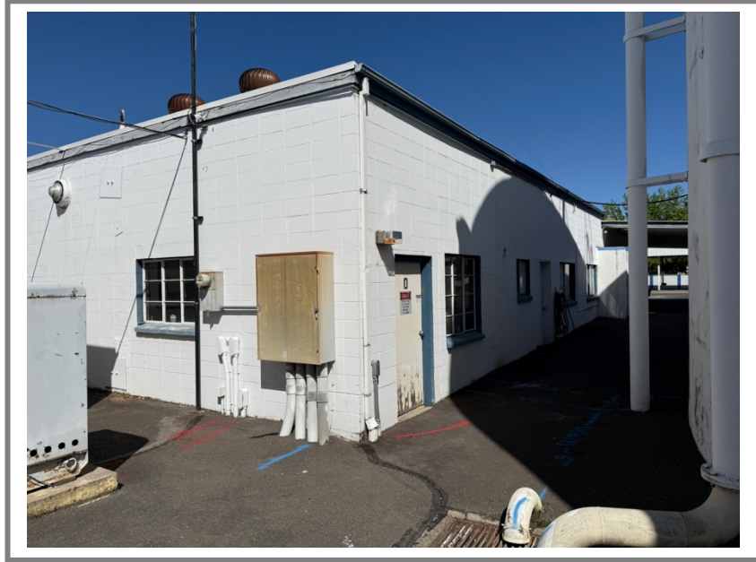
View toward side elevation and pump house room of north side shop building
