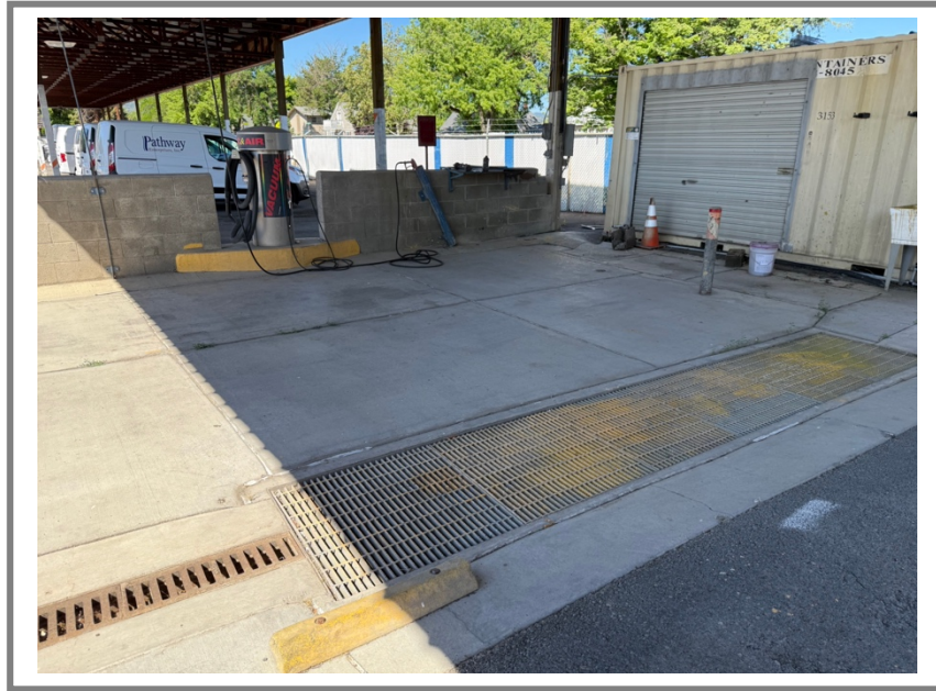
Views of car wash station with drain and grease catch on east side of canopy
