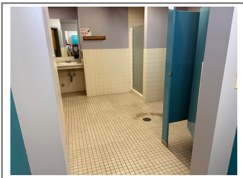
Interior view of men's restroom on first floor of office
