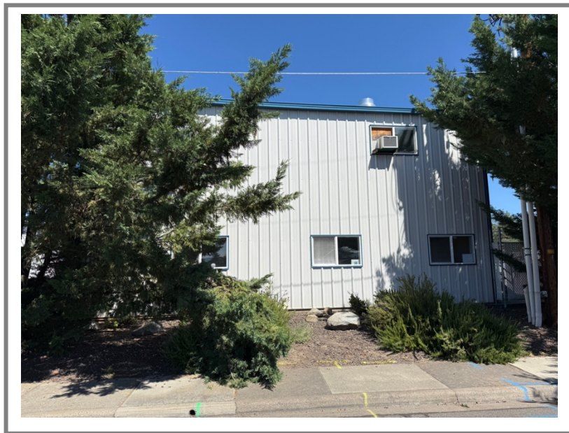
View of side elevation of office building from Cedar Street
