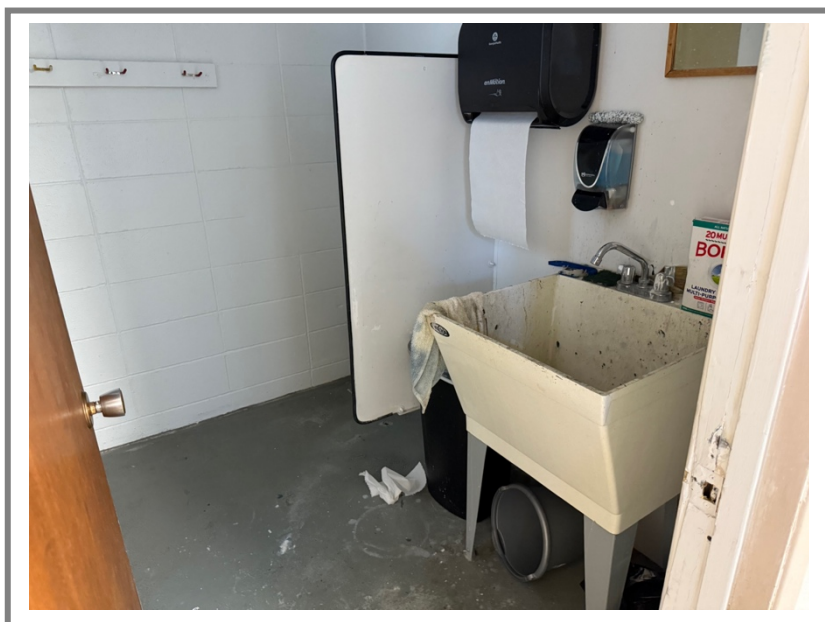
View of north side shop restroom
