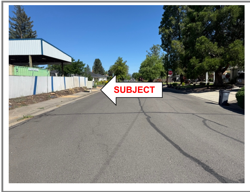
View north on Ashley Place at subject frontage
