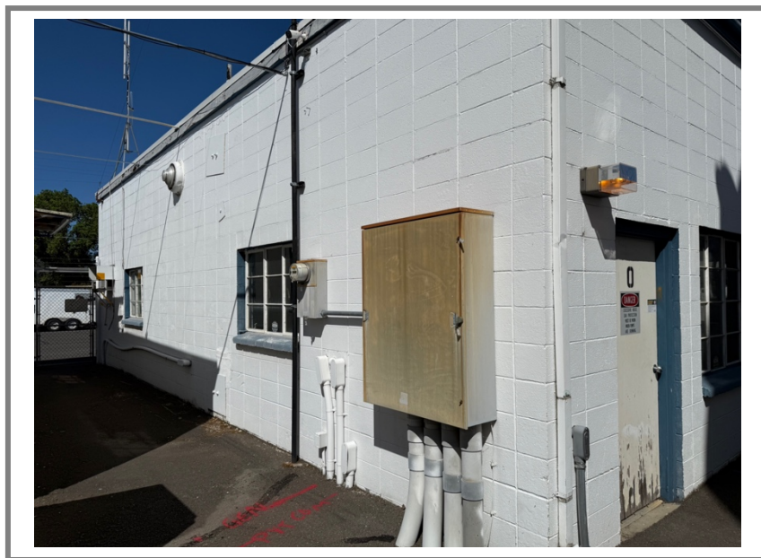
Rear elevation of south side shop building (Access)
