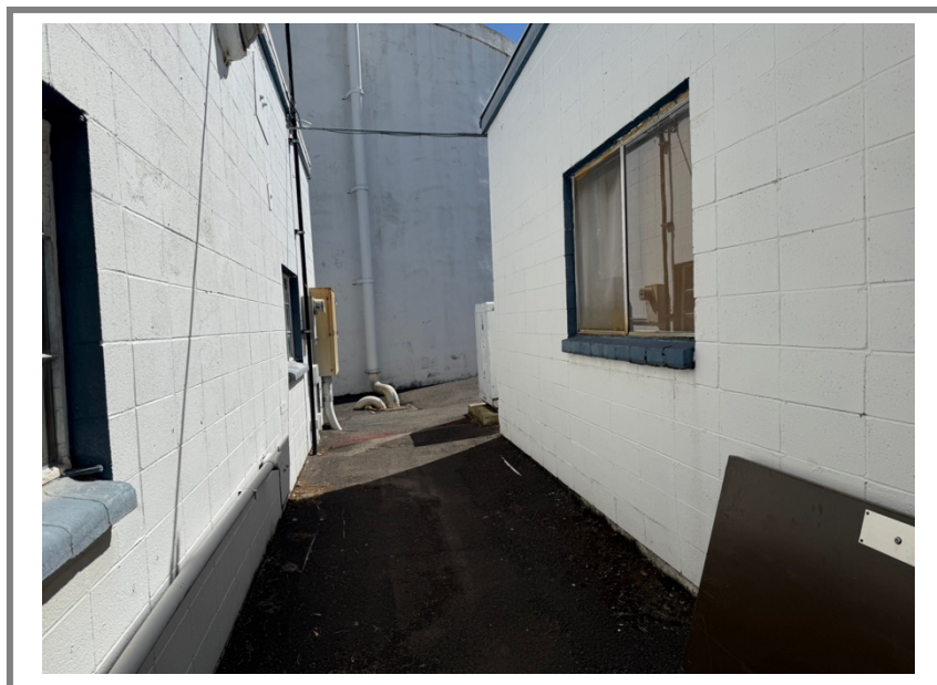
View of walkway between shop buildings
