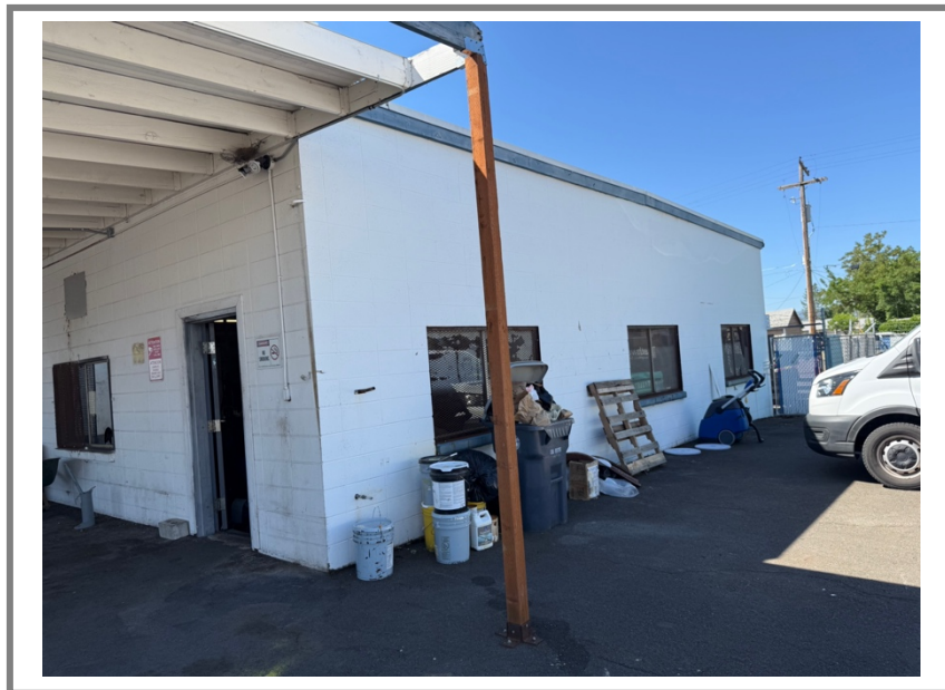
Side elevation of north side shop building (Pathways)
