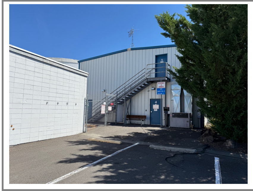
Views of main entry to office building
