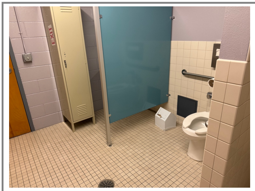
Interior view of women's restroom on first floor of office
