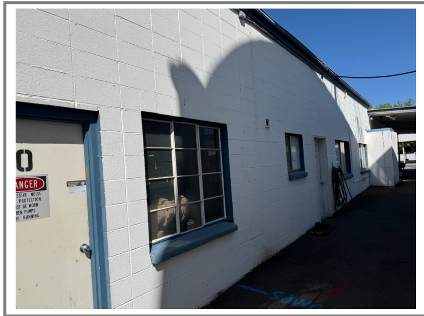
Rear elevation of north side shop building (Pathways)
