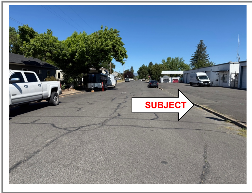
View north on Fifth Street at subject frontage
