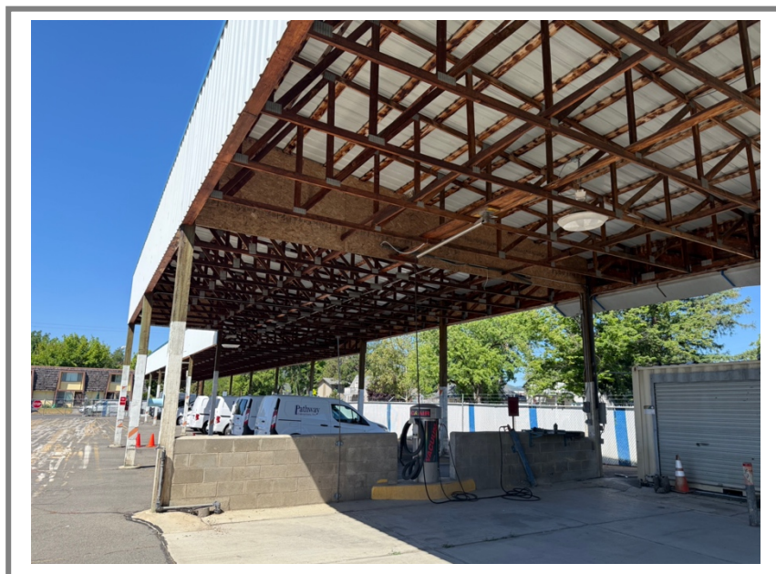
Views of parking canopy structure
