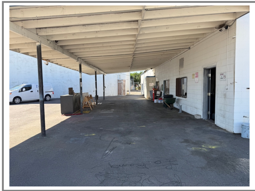
Views of canopy area on east side of north side shop building
