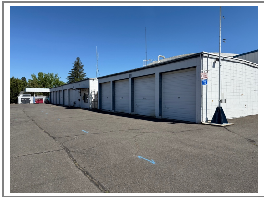
Front elevation of shop buildings from Fifth and Cedar Streets
