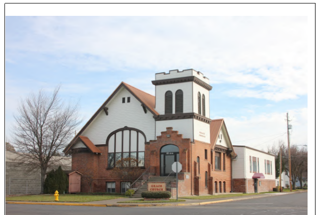
Looking SE from First St
