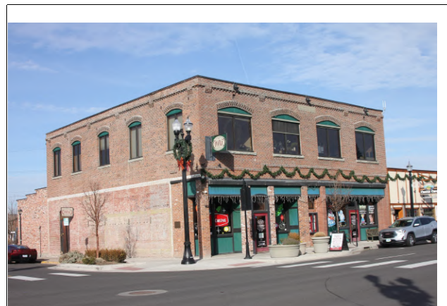
Looking NE from E Pine St
