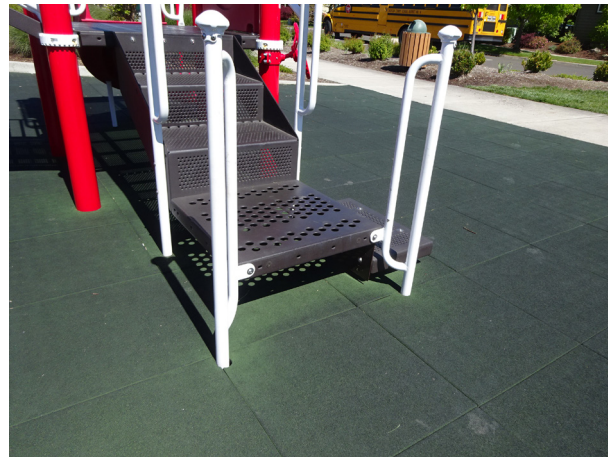
Figure 6. Play equipment transfer platform
