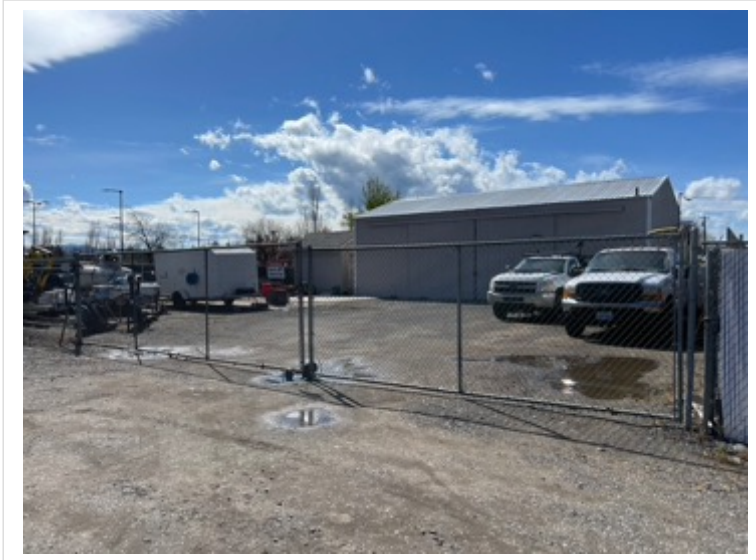
View of service commercial facility adjacent west of subject
